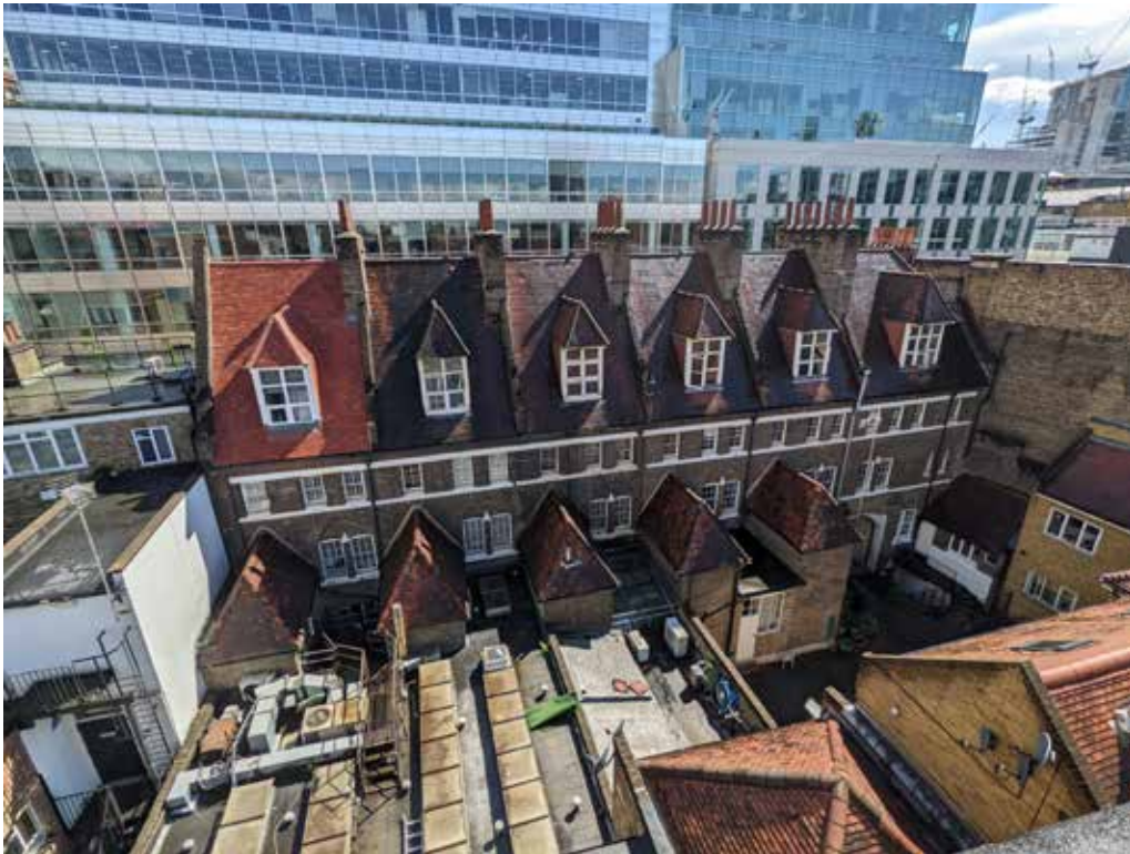
Existing Rear Infill Extensions
