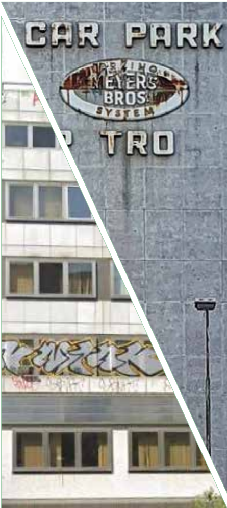
Curtain Road/ Worship Street
